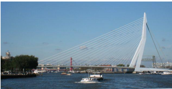
Rotterdam has used striking bridge design to open up areas for urban regeneration.
